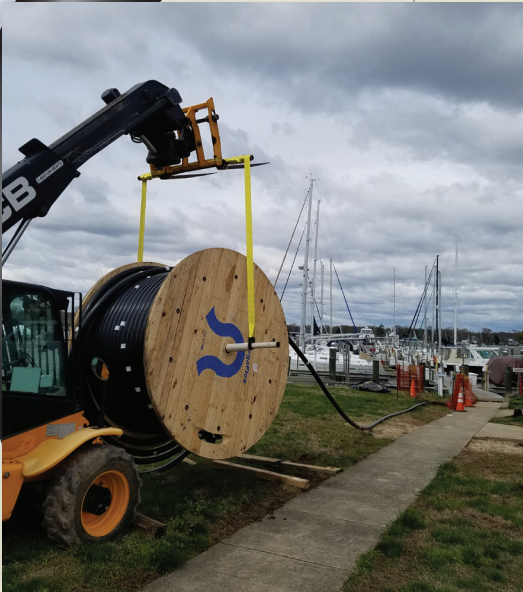
DoubleTrac is shipped on a robust 80" reel with a 3" arbor hole, allowing the pipe to be unrolled using normal construction equipment.
