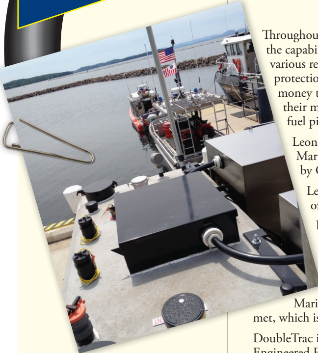
DoubleTrac's flexibility allows for easy installation into custom containment boxes.
