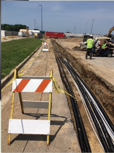
300ft trench with (5) runs of 2" DoubleTrac
