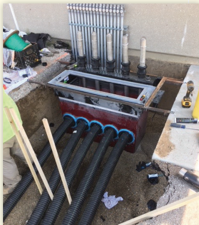
transition sump that will transition from 2" DoubleTrac to rigid piping.
