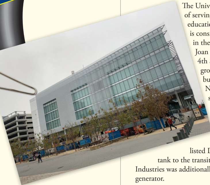
The Joan and Sanford I. Weill Neurosciences Building located 1651 4th St. Building 23A San Francisco, CA 94158.
