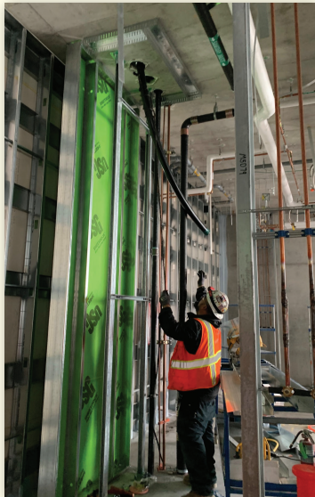
Routing DoubleTrac® piping between the floors of the building.
