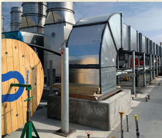
Southland employees unreeing the 1-1/2" DoubleTrac® piping (UGF-FSP-24) for the fuel oil supply line.
