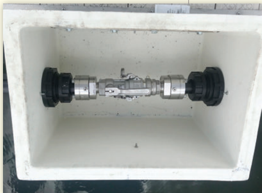
DoubleTrac transition sump with DoubleTrac removable entry fittings.
