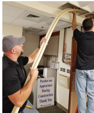
Pulls like wire through tight spaces with no fittings behind the wall or in the attic.
