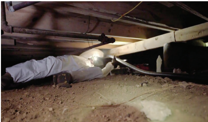
Pulls like wire through tight spaces with no fittings behind the wall or in the attic.
