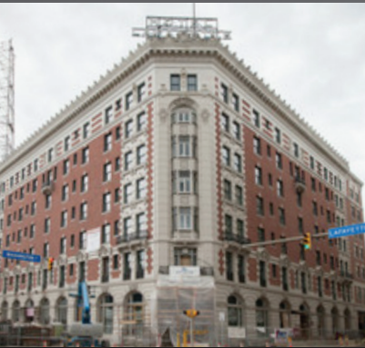
HOTEL TO APARTMENT CONVERSION
