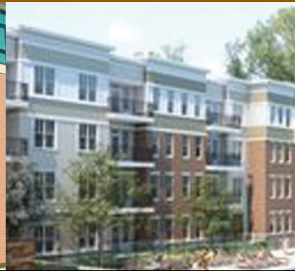
NEW CONDO INSTALLATION
