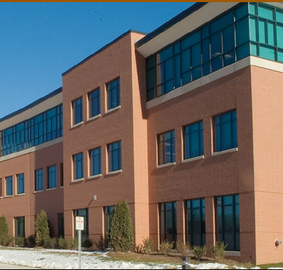
SCHOOL LAB INSTALLATION
