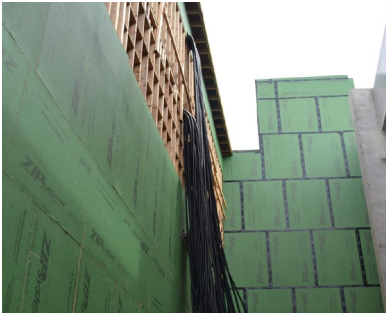
CounterStrike® install to appliance.
